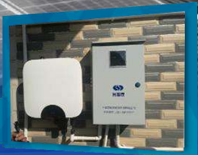
5.4kWp Residential PV System in Shanghai, China
