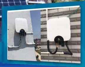
5.8kWp Residential PV System in Shanghai, China
