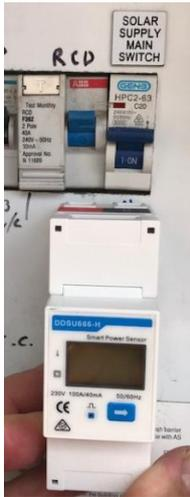
Pictured left, Huawei smart meter for single phase.
